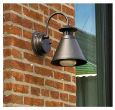
This light at the exterior of a building is shielded to limit spill-over lighting.
