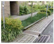
**Parkway with Infiltration:** A parkway set flush with the sidewalk allows stormwater runoff to collect in the planter area and infiltrate into the ground. Appropriate landscape material must be selected and overflow outlets provided.
