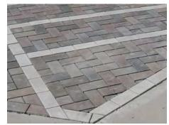
**Permeable Pavers Option 2:** Pavers set in herringbone pattern
