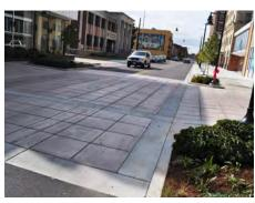
**Decorative Concrete Crosswalk:** Aggregate, color, and saw-cut lines create a durable decorative crosswalk. (Ensure that aggregate is flush if installed)
