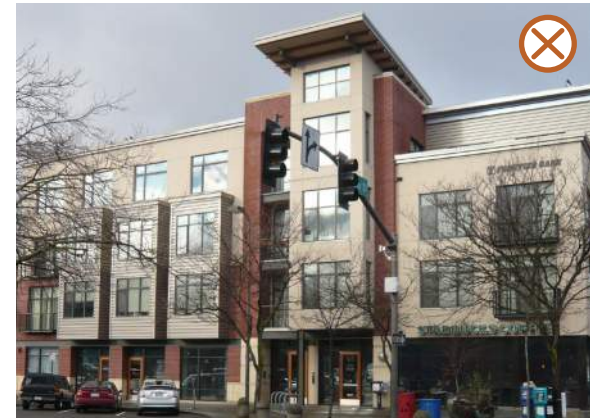
While third-story building components may be appropriate, fourth and fifth stories are inappropriate for Character Area 4.
