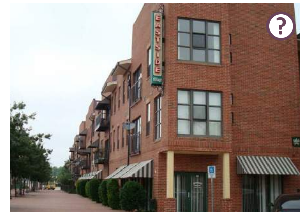
While the material and height are appropriate, breaking this building into more defined modules would be fitting.
