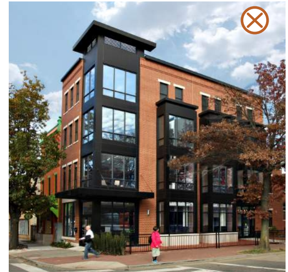
The height of this building is inappropriate for Character Area 5 but the use of materials and general style is appropriate.
