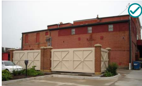
Minimize the visual impact of mechanical equipment from the public right-of-way using screen walls or other screening methods.
