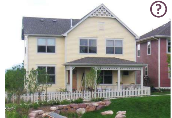
While this residential building exhibits traditional features, its lack of setback and minimal space between the neighboring home is inappropriate for Character Area 9.
