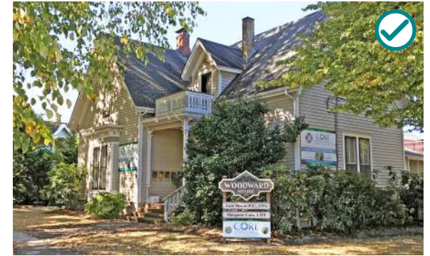
Adaptive reuse of a residential structure to an office space, maintaining the original features of the structure
