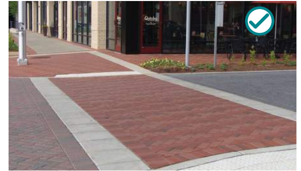
Visually distinguish pedestrian crosswalks.
