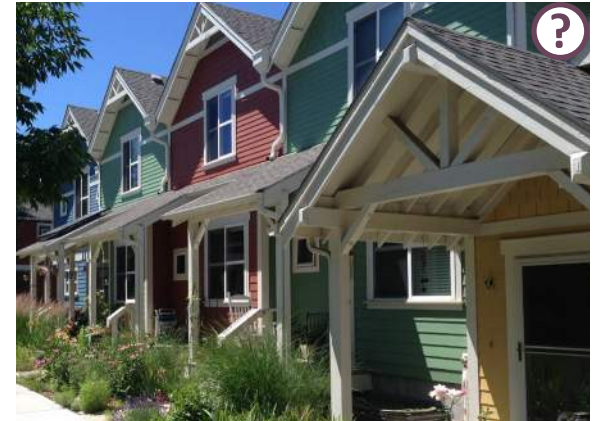
While the gable roof form and scale of these residential townhomes is appropriate, brick and more muted colors would be more appropriate.
