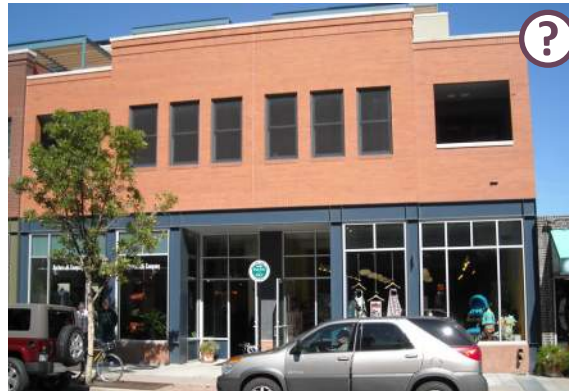
While the materials are appropriate, setting the second story back from the property line to prevent a sheer wall would be better.
