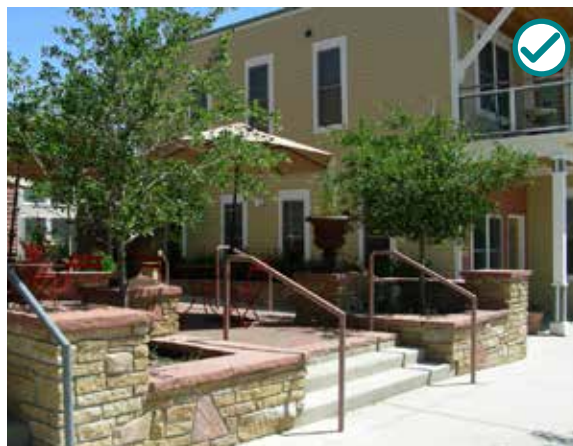
Consider incorporating private outdoor space to enhance new uses. This patio provides an opportunity for café patrons to sit outside.
