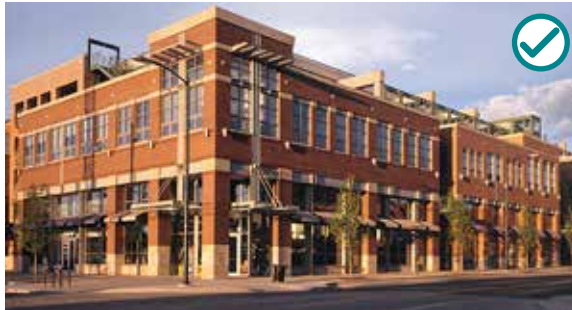
The scale and materials of this building are appropriate.
