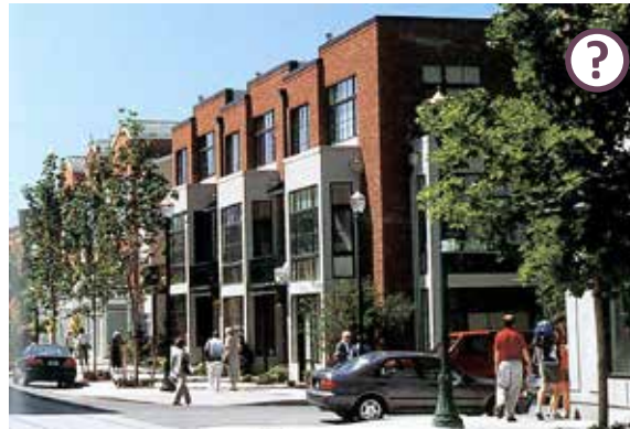
While this townhome is an appropriate height, breaking the building into smaller modules would make it more appropriate.
