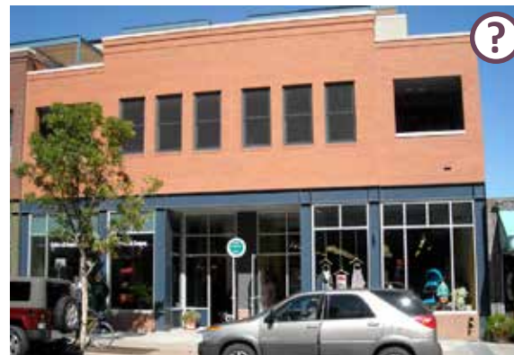
While the materials are appropriate, setting the second story back from the property line to prevent a sheer wall would be better.
