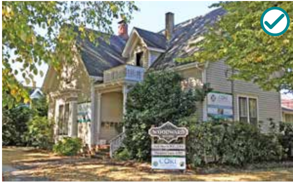
Adaptive reuse of a residential structure to an office space, maintaining the original features of the structure
