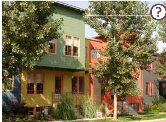
The "artistic" quality of this building is appropriate, but the scale may be too large.
