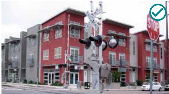
A mix of materials and clear entry definition make this mixed use building appropriate.
