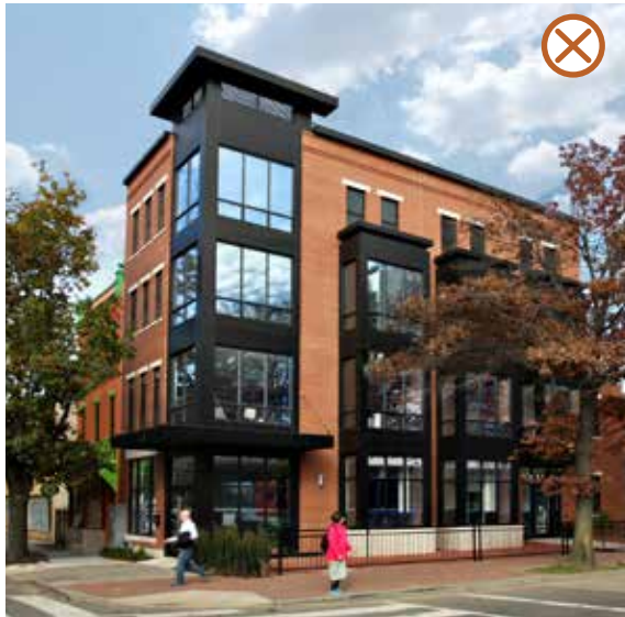
The height of this building is inappropriate for Character Area 5 but the use of materials and general style is appropriate.
