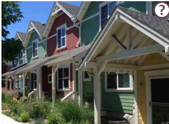
While the gable roof form and scale of these residential townhomes is appropriate, brick and more muted colors would be more appropriate.
