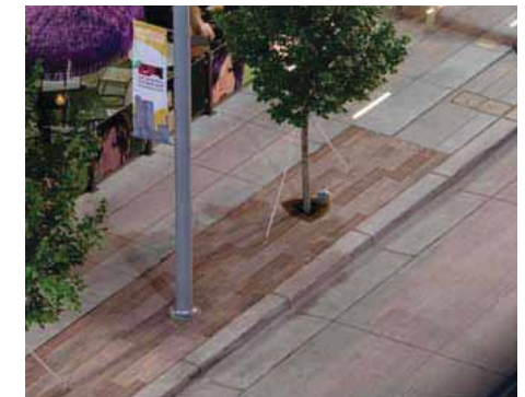
Inground Planter with Paving Installed
