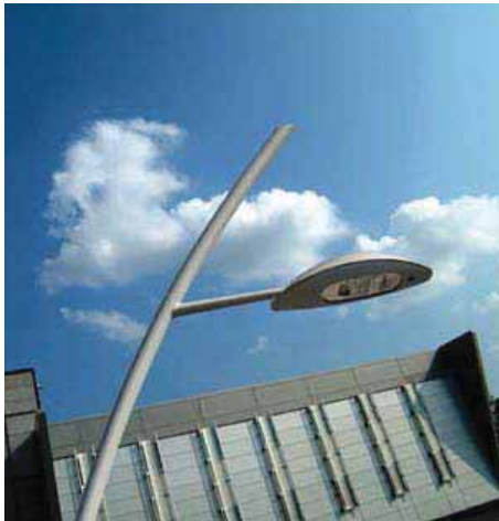
Full cut-off Full cut-off optics protect the night sky.
