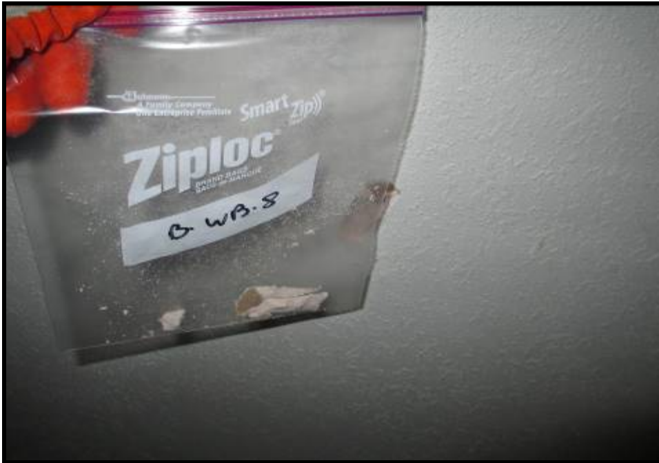
Photo 10: South Unit Bath Drywall
