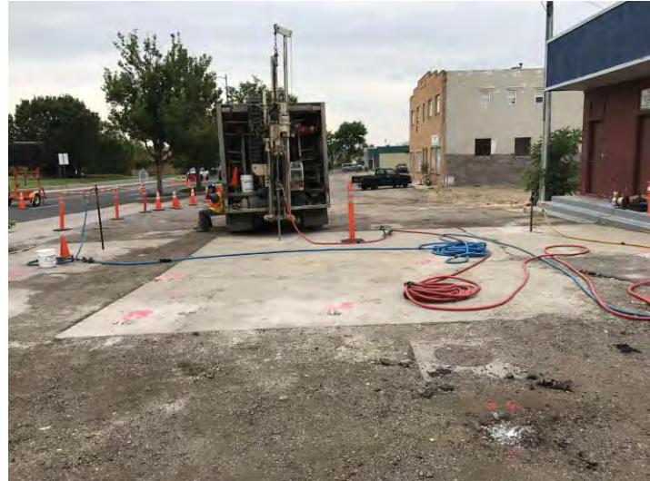
Between July 11 and 21, 2017, CGRS subcontracted Regenesis Remediation Services (RRS) to perform PersulfOx, RegenOx, and ORC-A injections on- and off-site (7287 Lowell Boulevard) via direct push in the locations that were potholed and backfilled as mentioned above. The following table provides a summary of the injections in each of the five areas:
