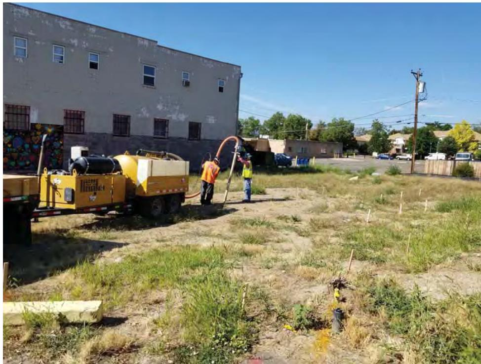
Photo 3 .Potholing injection points in the field south of the building located at 7287 Lowell Blvd. 8/28/2019
