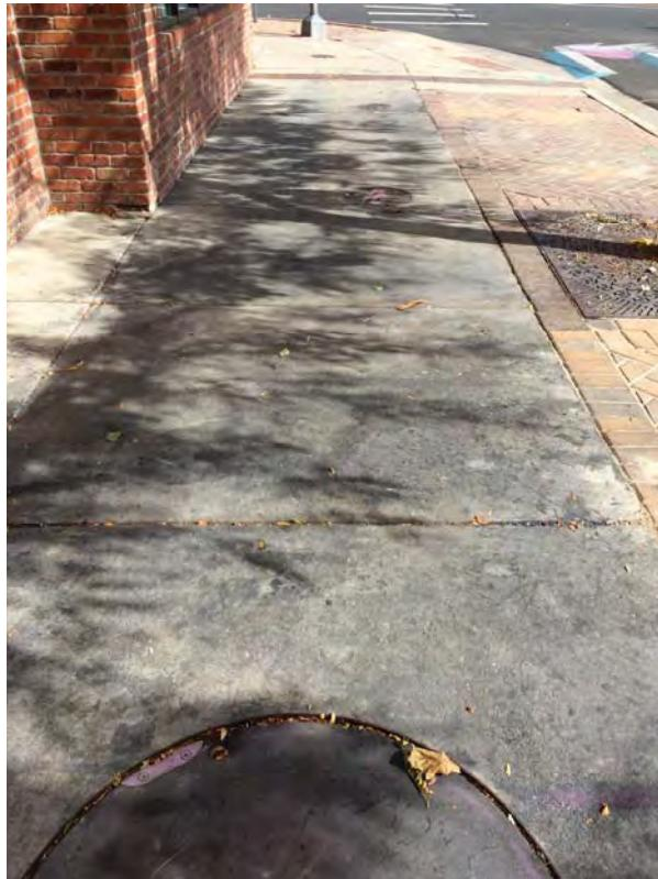
Photo 11. Carbon staining on sidewalk in front of 7305 Lowell Blvd. These sidewalk panels will be removed when remediation and monitoring wells are decommissioned.
