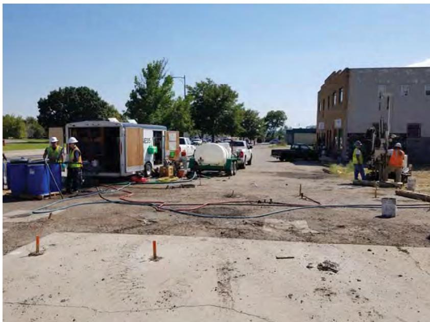
Photo 6. Injecting in multiple injection points, mixing PetroFix™ injectate, and direct pushing new injection points at 7287 Lowell Blvd. 9/17/2019
