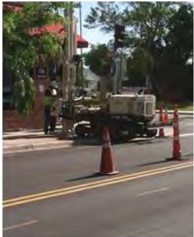
2,400 gallons. The injection was performed at an average pressure of approximately 26 psi with an average flow rate of approximately 4 gpm. The injection interval ranged between 9 and 17 feet bgs.
